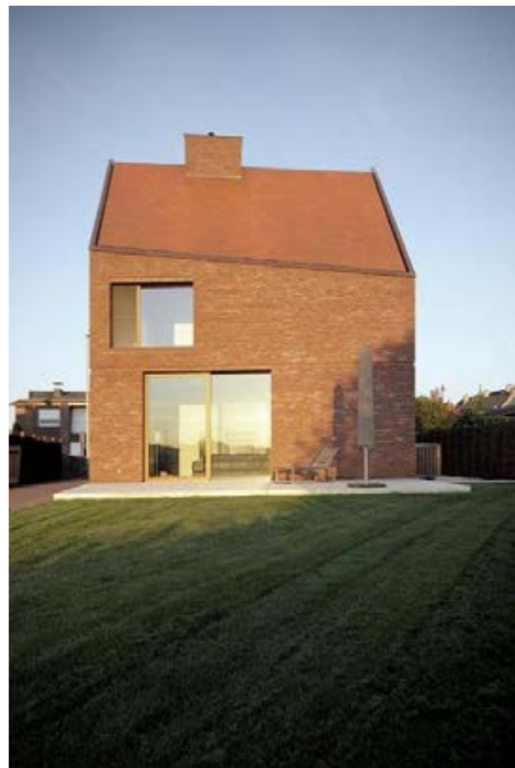
RE-ST Architecten, Belgium
