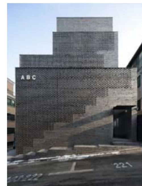
ABC Building, Wise Architecture, South Korea
